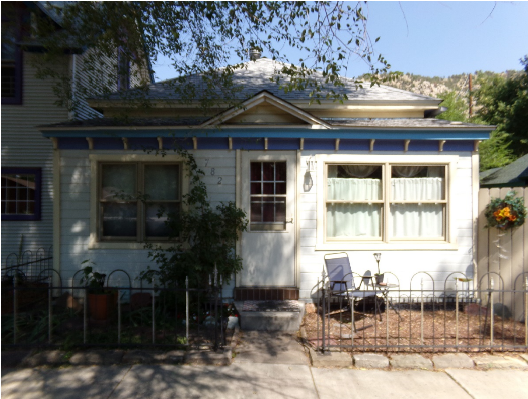
Photo Number: 5GF.5893_1 Description: Looking at the primary (south) elevation of the building. Date: 9/6/2022 View: North
