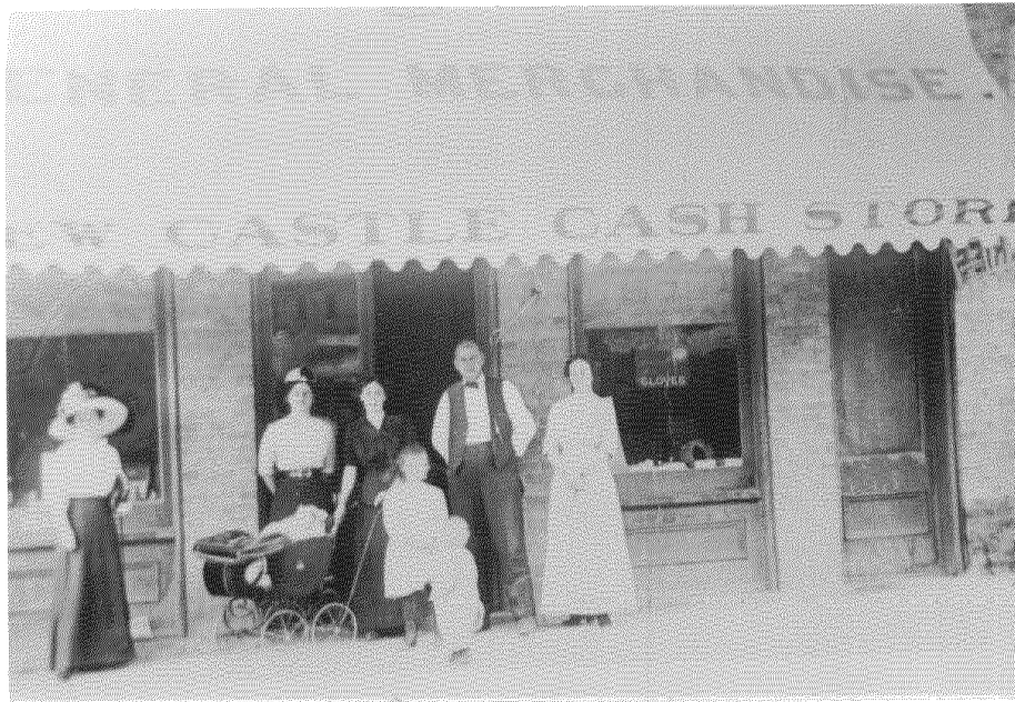
The New Castle Cash Store was located on the lower floor of 500 W. Main Street. SOURCE: Steve Rippy, photographic collection.
