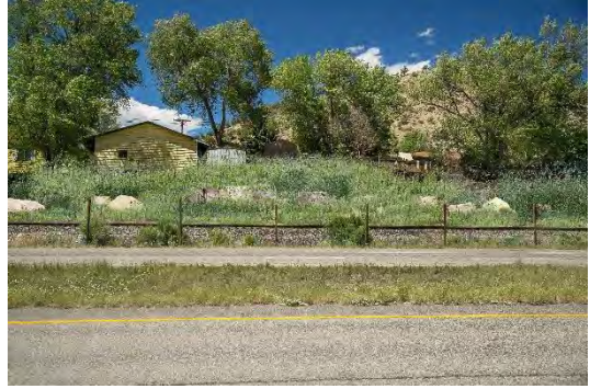
Possible Future Hillside Repair
