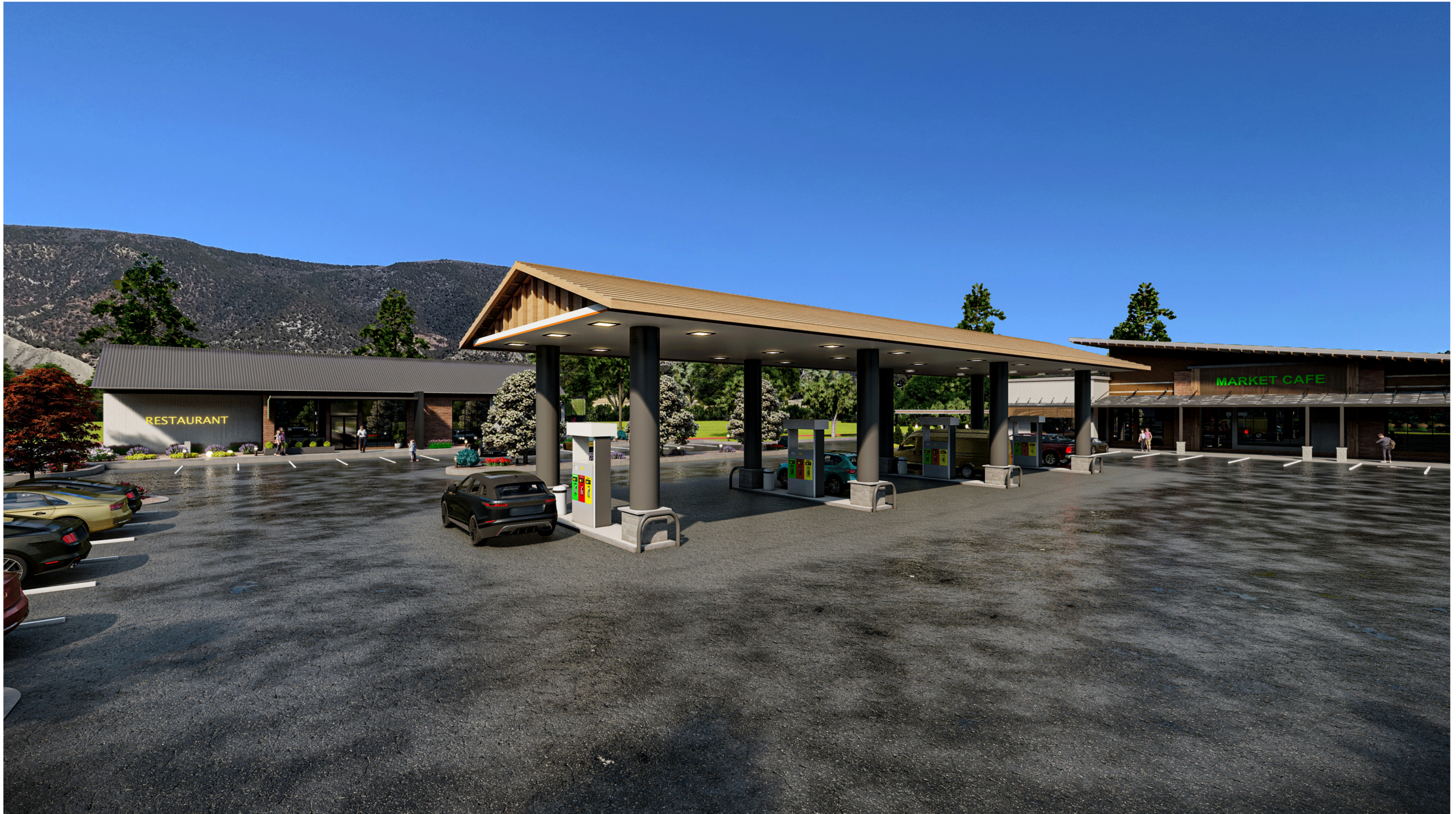
View F - Fuelling Shed/Gas Station
