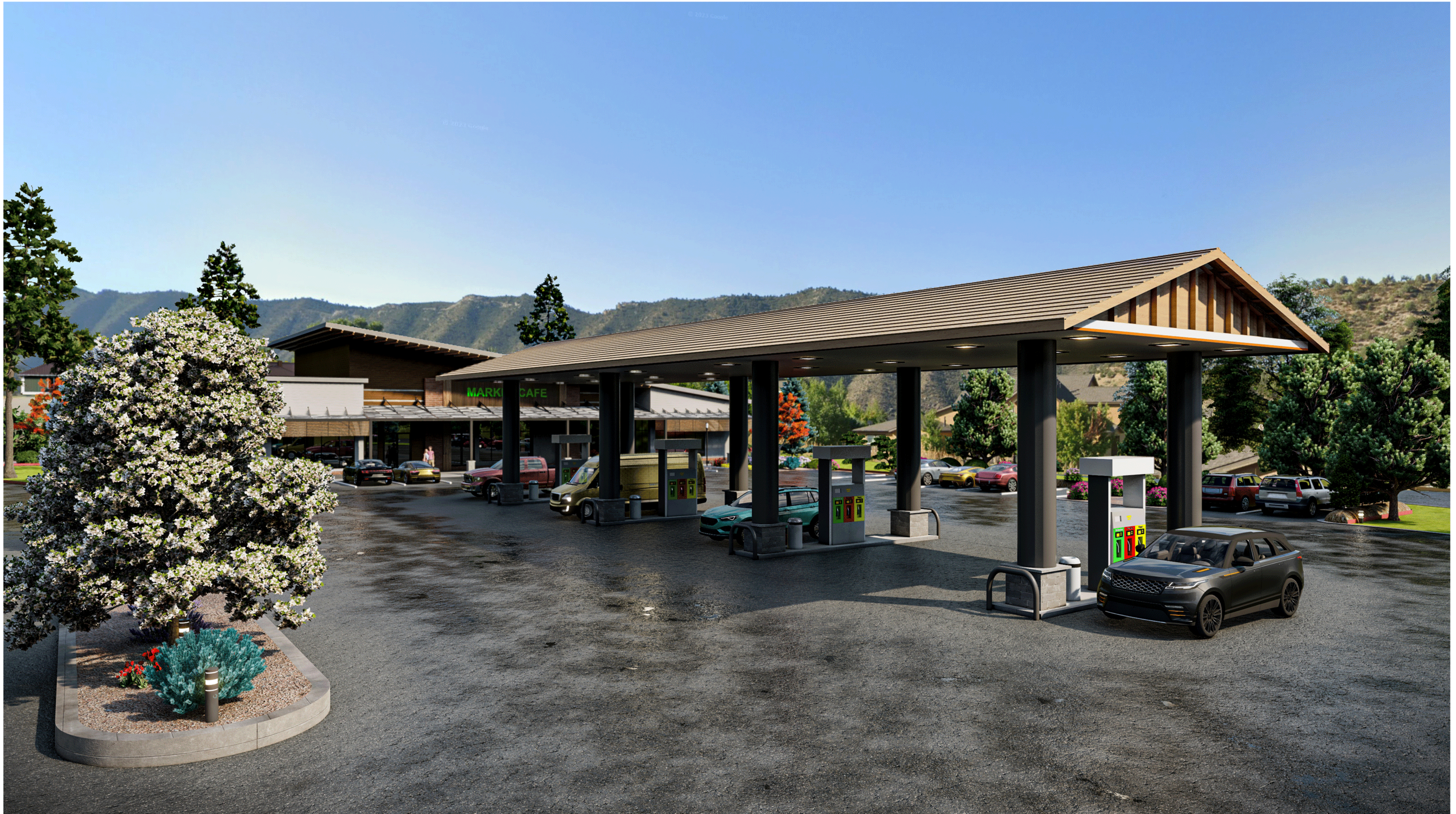
View G - Fuelling Shed/Gas Station
