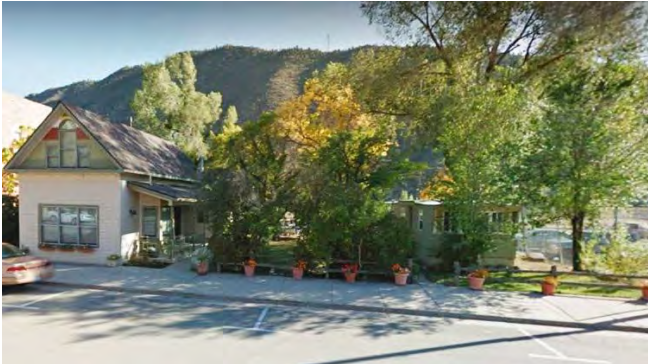
Mobile Home adjacent to Single Family Residence
