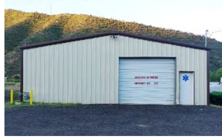
Vacant Metal Building
