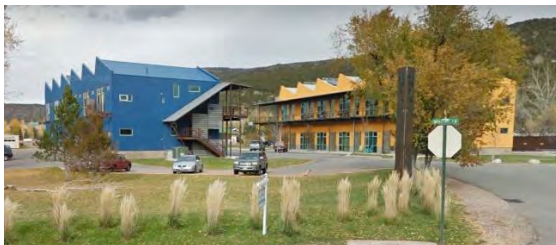
Mid-Valley Design Center Live-Work
