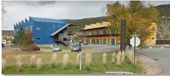
Mid-Valley Design Center Live-Work
