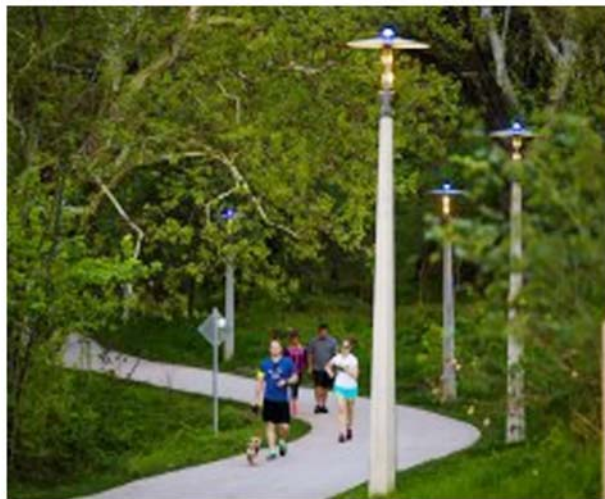
Pathway lighting added to encourage evening and night use and for safety
