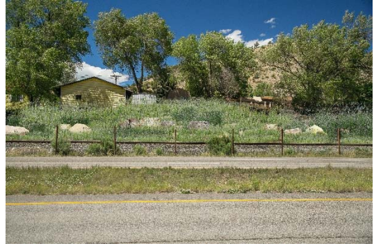
Possible Future Hillside Repair
