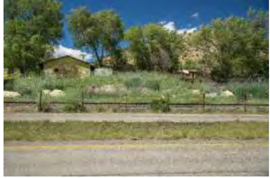
Possible Future Hillside Repair
