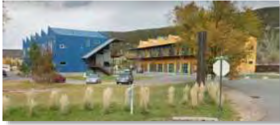
Mid-Valley Design Center Live-Work
